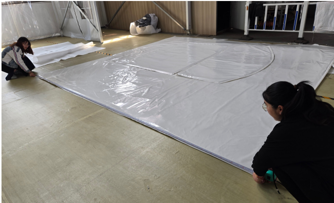
PVC cover inspection and dimension checking
